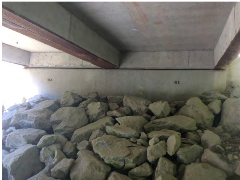
Right Bank Abutment when facing downstream
