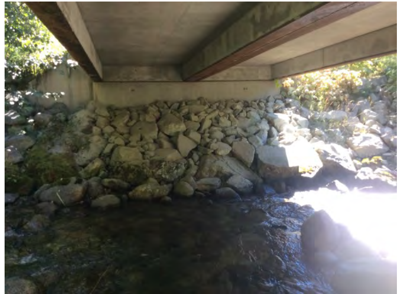
Left Bank Abutment when facing downstream
